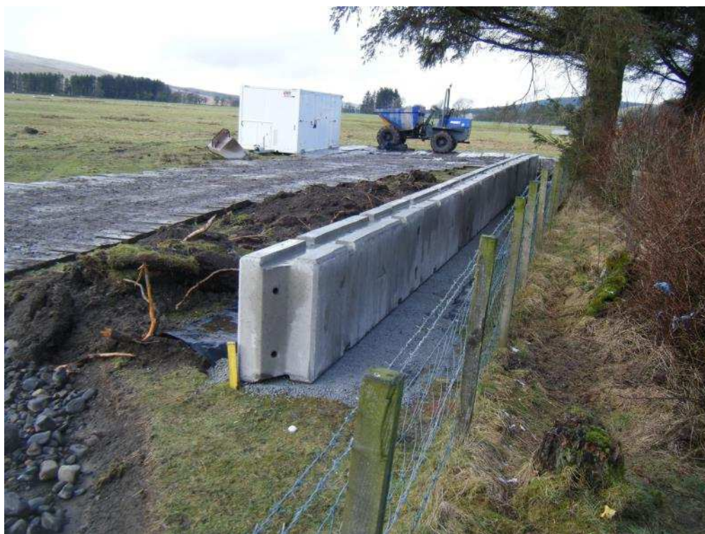
Photograph 5.2: Flood barrier under construction at Carsphairn
