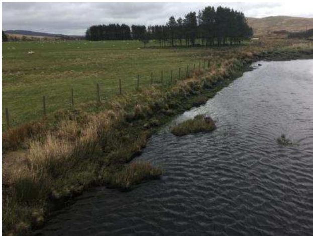
Photograph 7.5: Broad floodplain at Carsphairn with evidence of stock control measures
