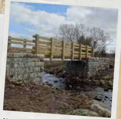
New Loch Skerrow footbridge created
