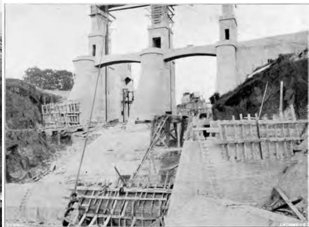
FIG. 22. FLOODGATES AND APRON; TONGLAND DAM.
