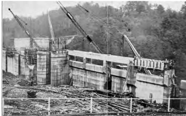
FIG. 118. EARLSTOUN DAM UNDER CONSTRUCTION.
