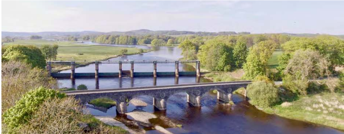
GLENLOCHAR BRIDGE with Hydro Scheme Barrage in background
