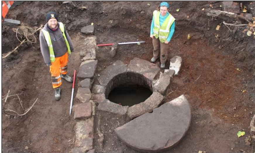
View of the Levensgrove well after excavation
