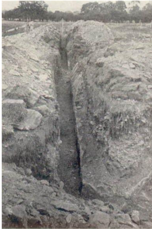
Wall chasing trench from 1911
