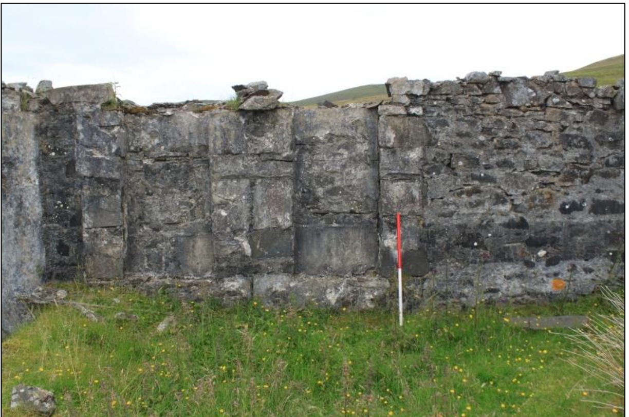
Figure 10b: Building [003] – blocked windows at the south end of the west wall of Room B
