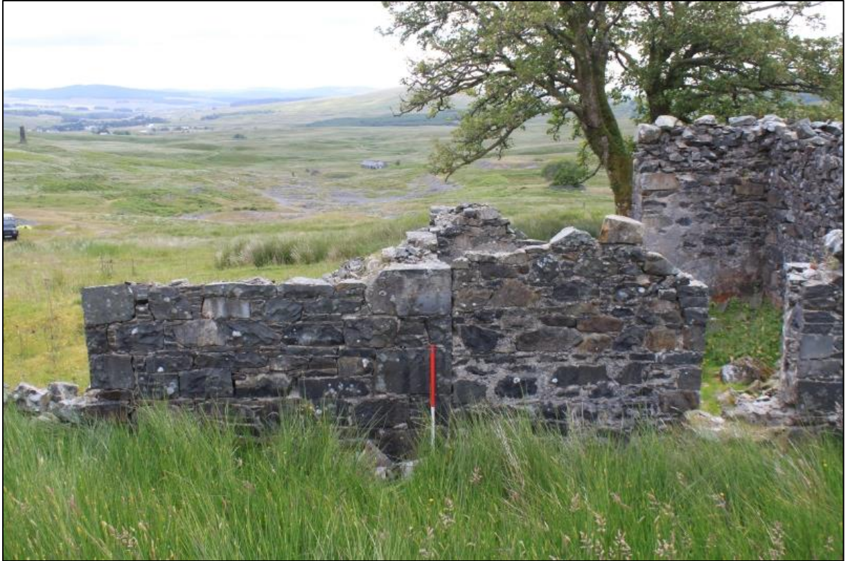
Figure 7a: External NW facing elevation of Building [001] showing junction between Rooms D and E
