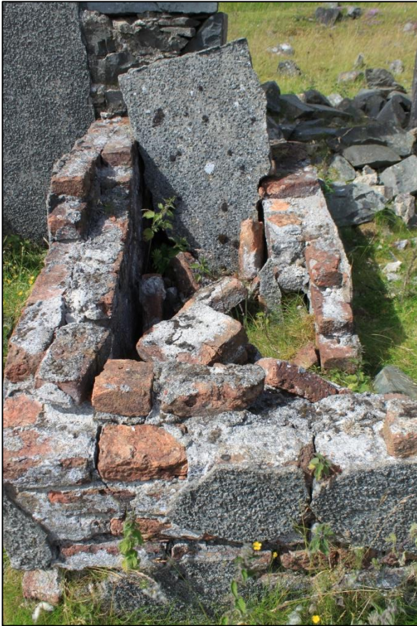
Figure 18a: Building [007] – SW end of Room E taken from the SE
