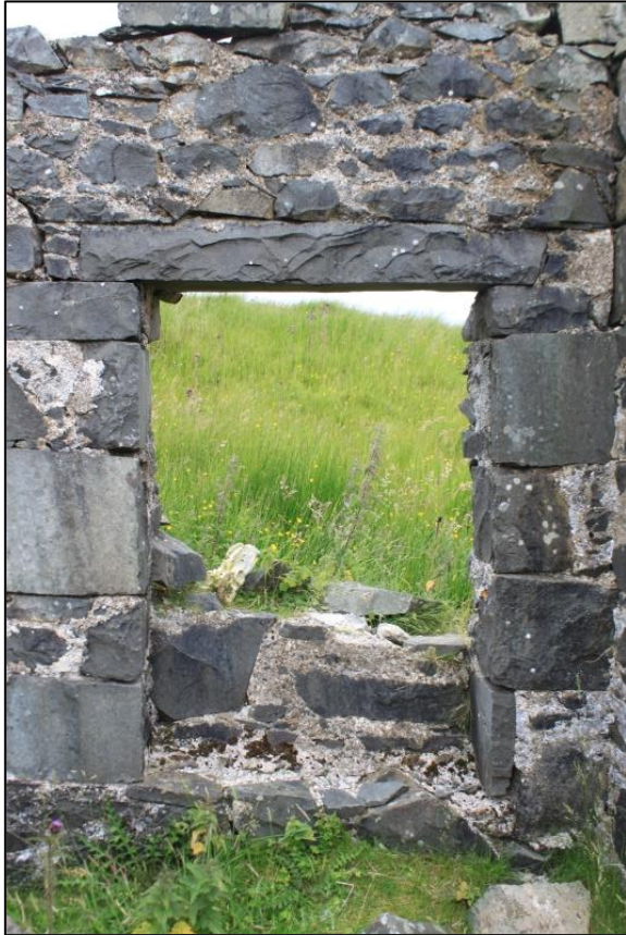
Figure 11a: Building [003] - partially blocked window in N wall of Room B
