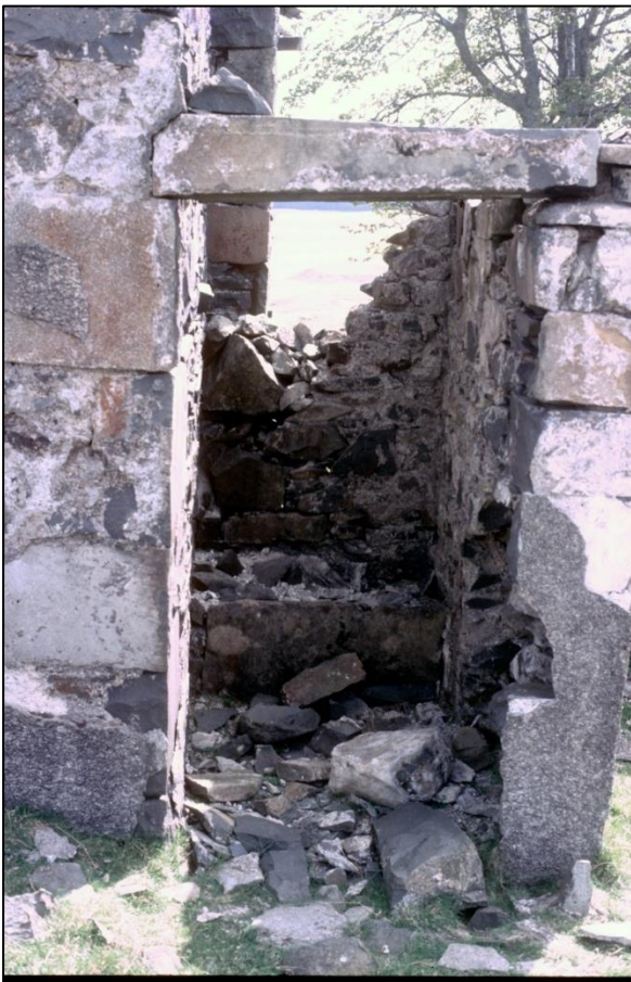
Figure 19b: Building [001] – external view of doorway in NW wall of Room A taken in 1987, courtesy of Anna Campbell
