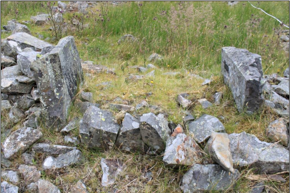
Figure 14a: Building [005] – possible jambs of fireplace in NE wall of Room C, taken from the SW
