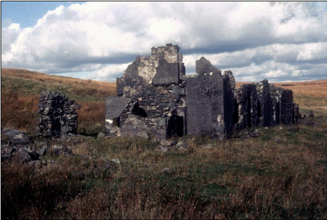
Figure 19a: View of Building [001] in 1993 taken from the southwest, courtesy of Anna Campbell
