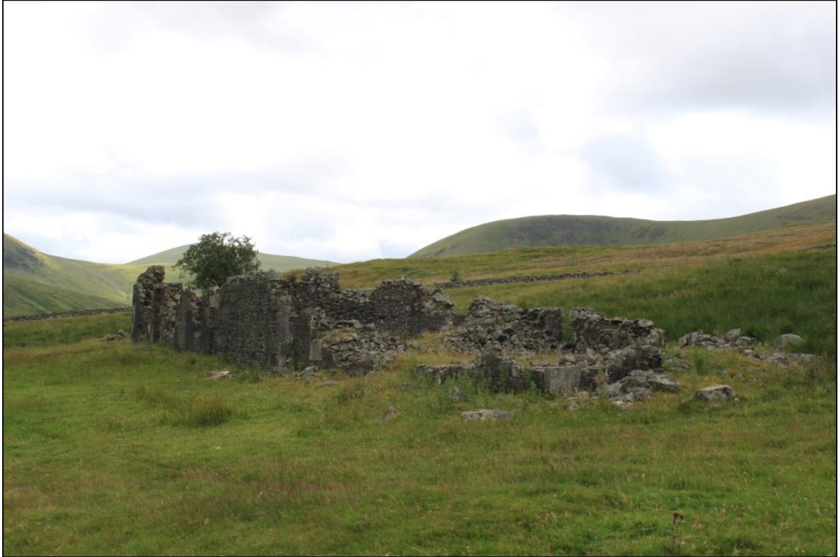
Figure 3a: General view of Building [001] from the northeast
