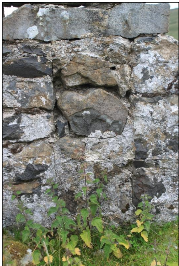
Figure 11b: Building [004] – blocked opening in SE wall
