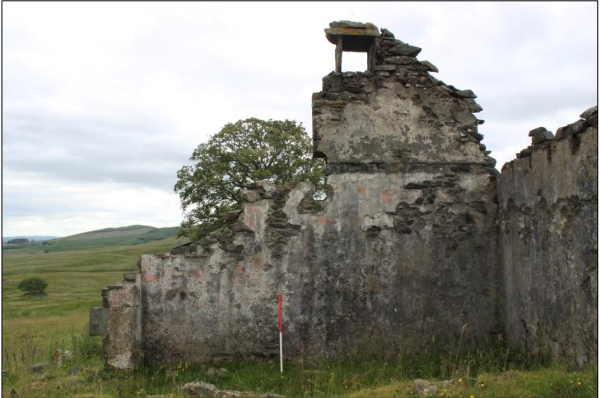
Figure 10a: Building [003] – south wall of Room A
