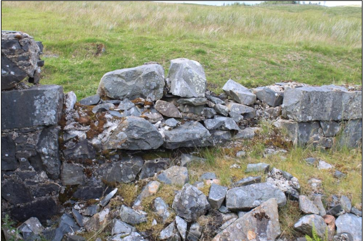
Figure 17a: Building [007] - blocked opening within NW wall of Room B, internal view
