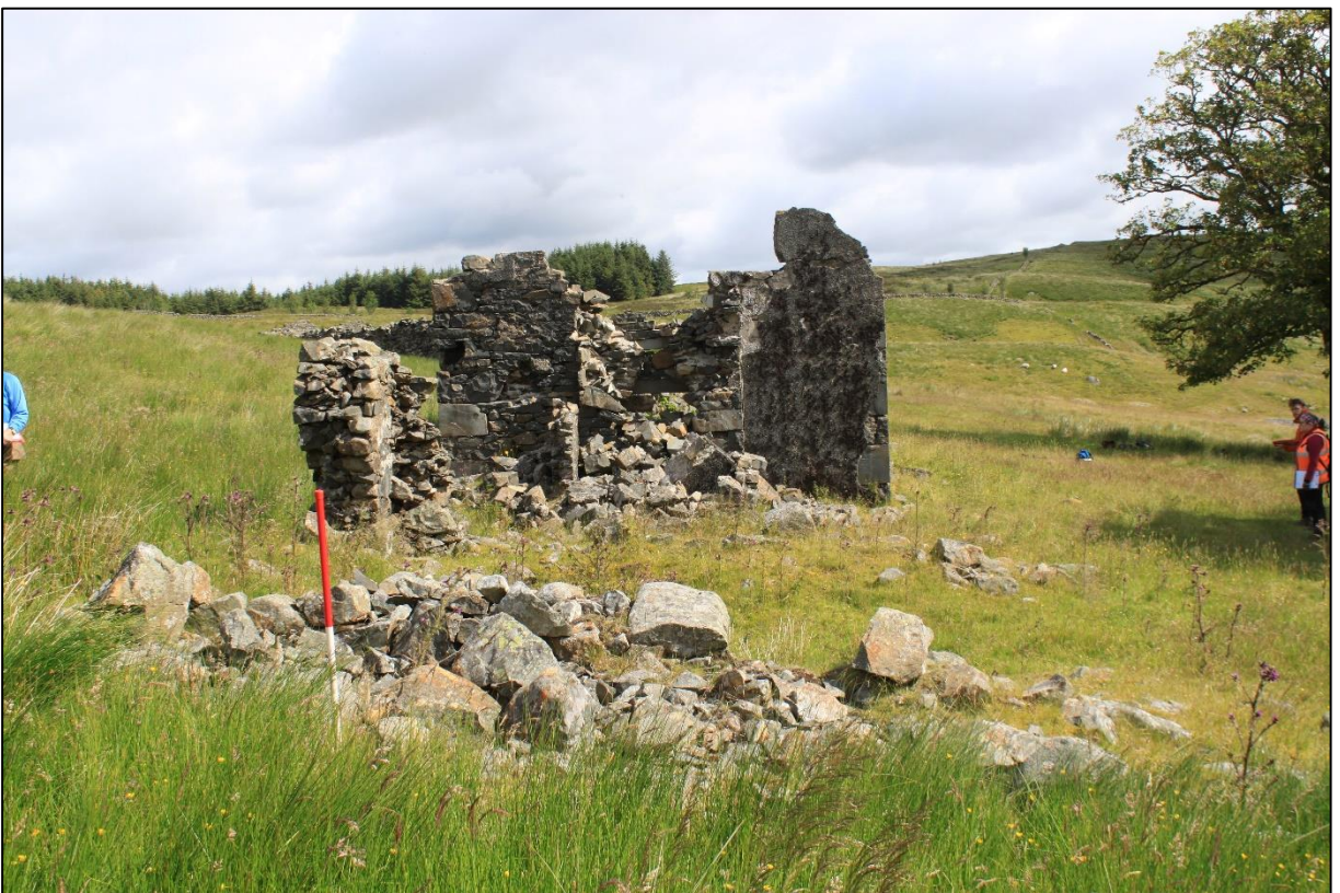
Figure 7b: General view of Building [002] from the southwest
