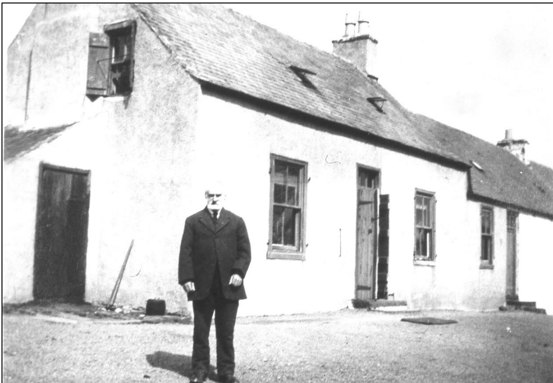
Figure 18b: 'David McMath at the leadmines September 1926' showing SW end of Building [001], image courtesy of Carsphairn Archive (see References)
