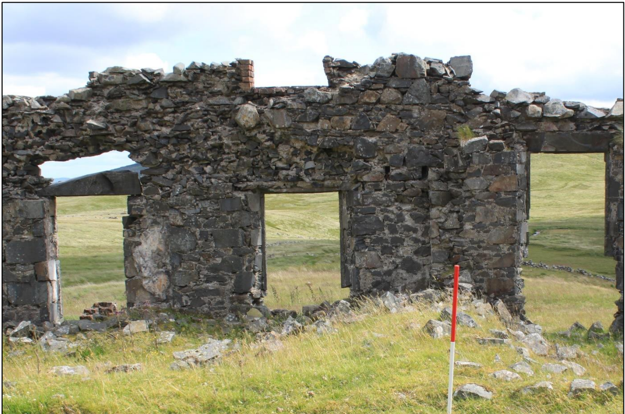
Figure 17b: Building [007] – Internal view of SW wall of Room D showing joist holes and brick traces around possible first-floor window
