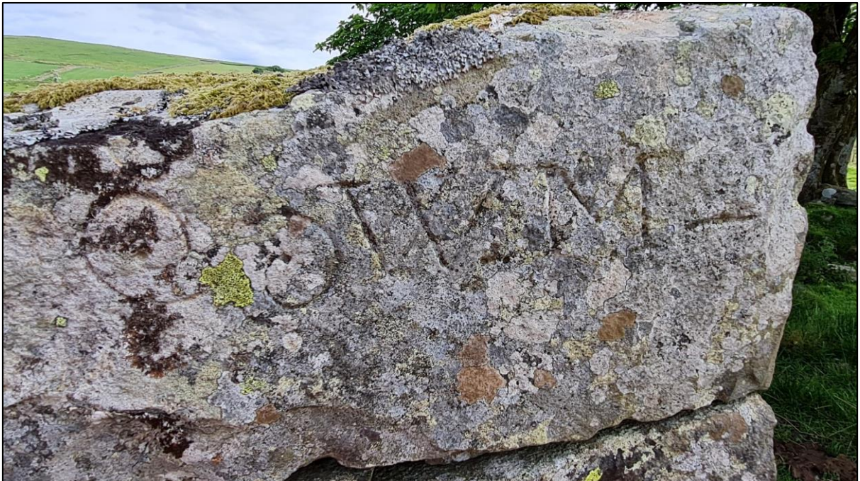
Figure 7b: Letters carved into a quoin in the external southwest facing elevation of building [1004], taken from the southwest
