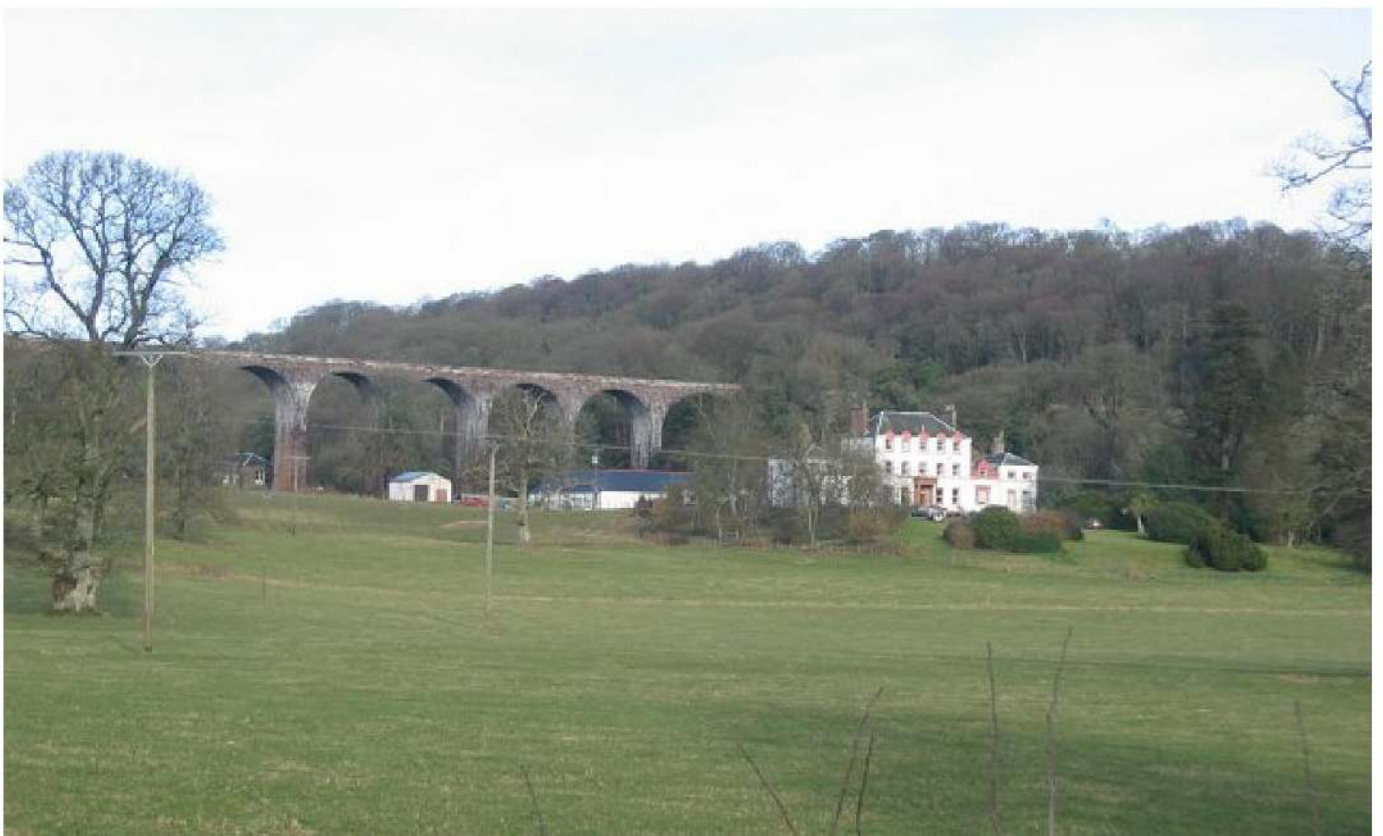
Viaduct as present.
