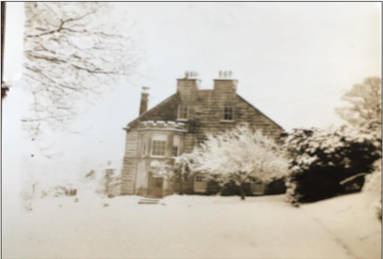
Figure 2: Janefield House. South Elevation, early 1950s
