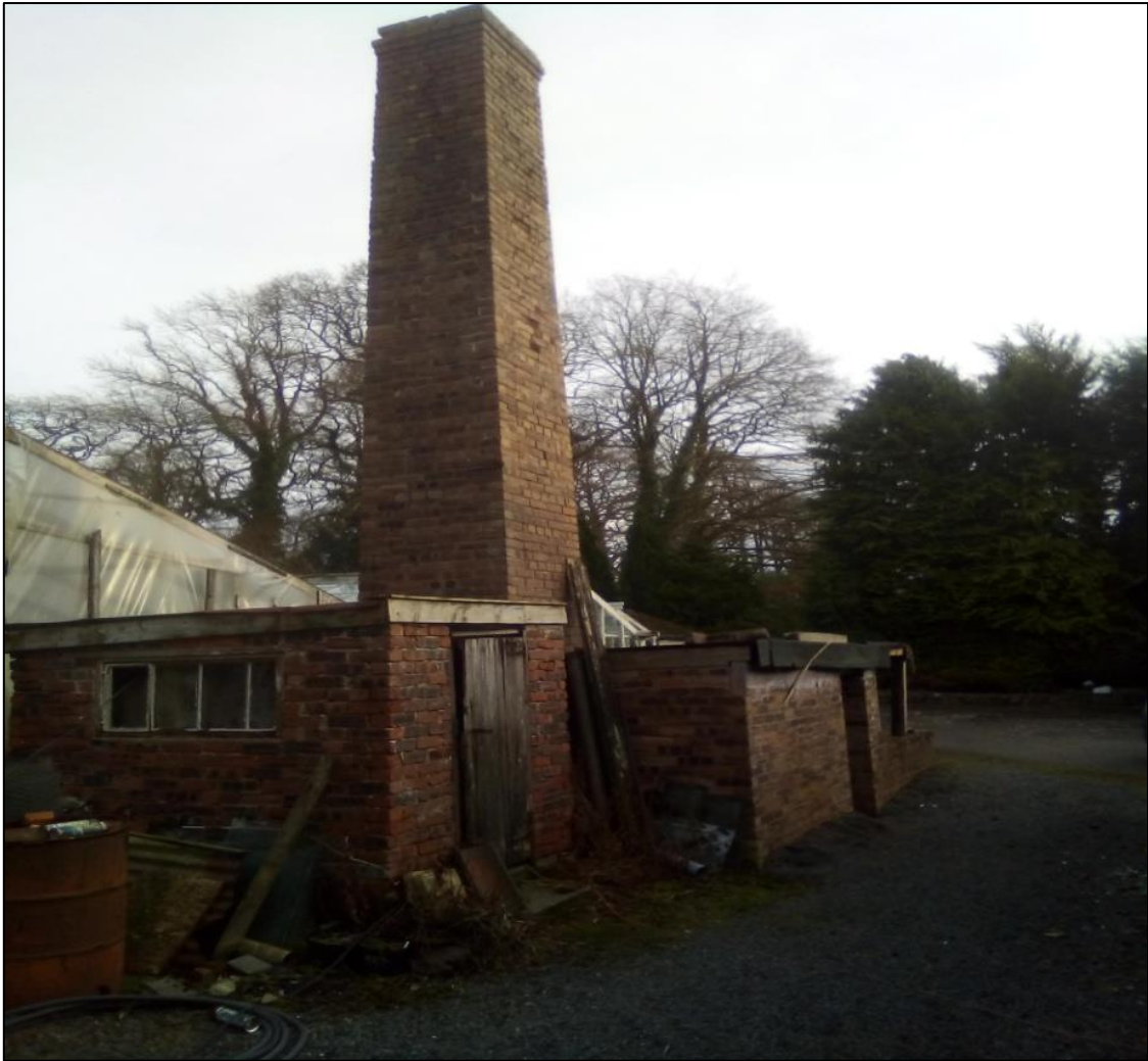
Figure 3: Remains of Heating System for the Greenhouses
