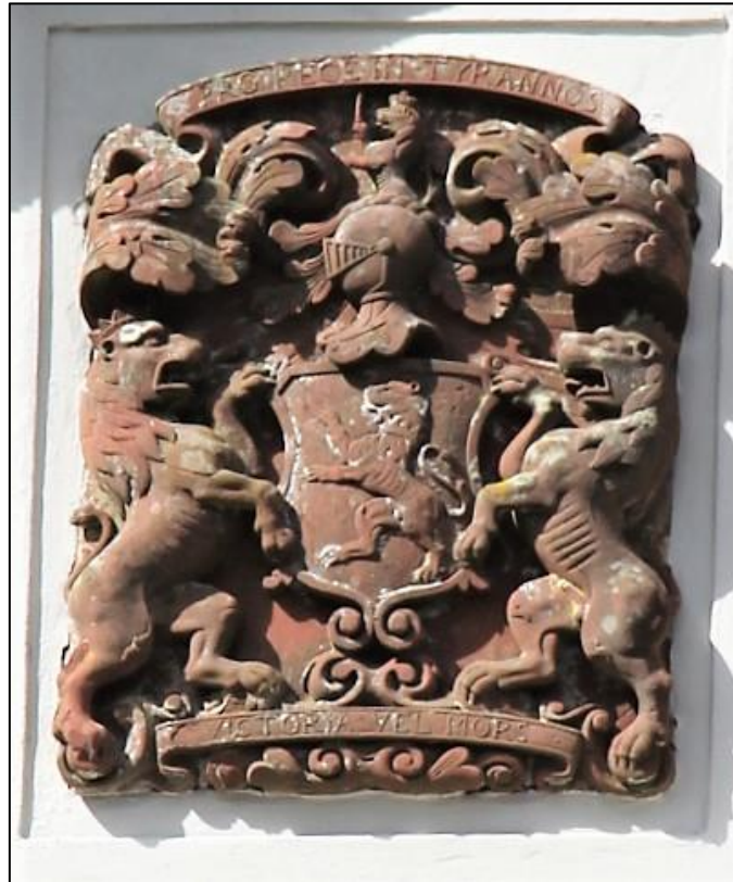
Red sandstone armorial plaque showing the McDouall arms incorporated into the east front. This plaque may have come from the 19th century additions to Logan House or from an earlier building.
