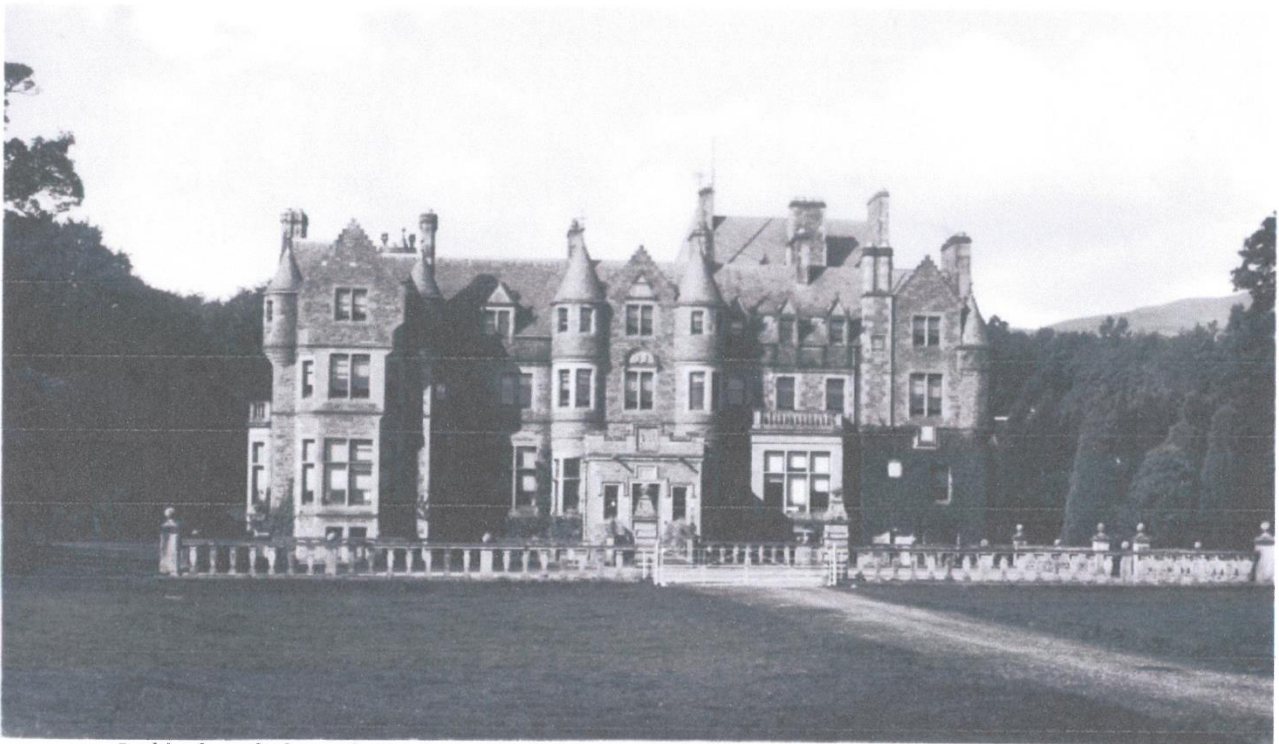
In this photo the lower floor at the extreme right appears to have vegetation covering a large section of wall.
