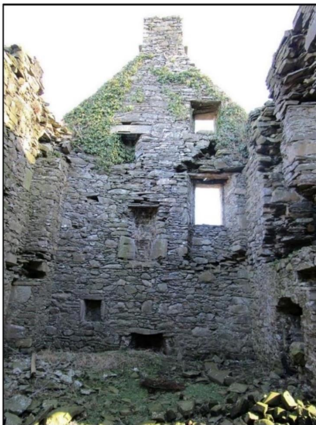
Figure 13: Interior, ENE Wall (WSW-Facing), Showing Fireplaces and Window Embrasures
