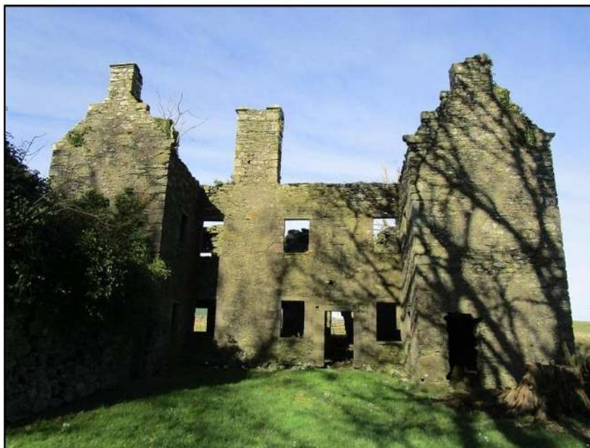
Figure 11: View of Front (ESE) Elevation
