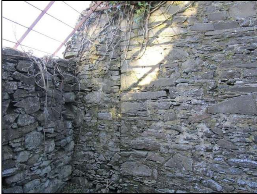
Figure 17: NNW Wall of Chamber 5, Showing Junction Between Original and Later Masonry
