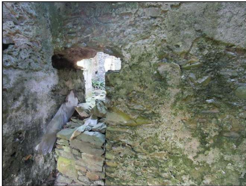
Figure 19: Partially blocked doorway linking Chamber 1 with Chamber 3 (ENE Wing), Viewed from Interior of Chamber 3
