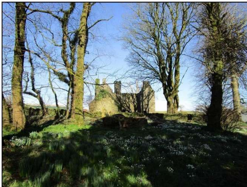
Figure 10: Borgue Old House in Wider Setting
