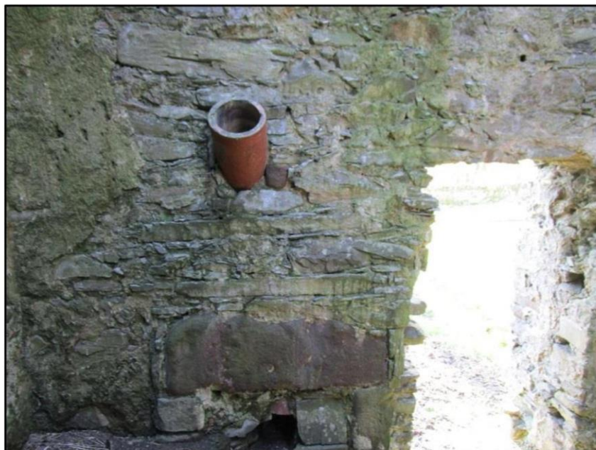
Figure 15: Inserted Opening and Ceramic Pipe in SSE Wall of Chamber 3 (ENE Wing)
