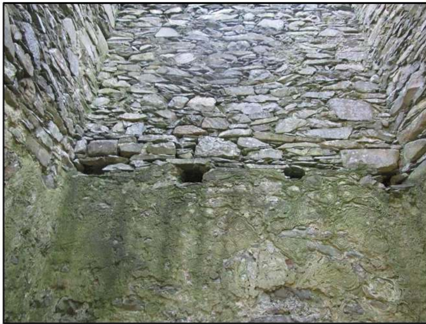
Figure 16: Joist-holes Marking Line of 1 st Floor Level with Plastered Wall Below, ENE Wall, ENE Wing
