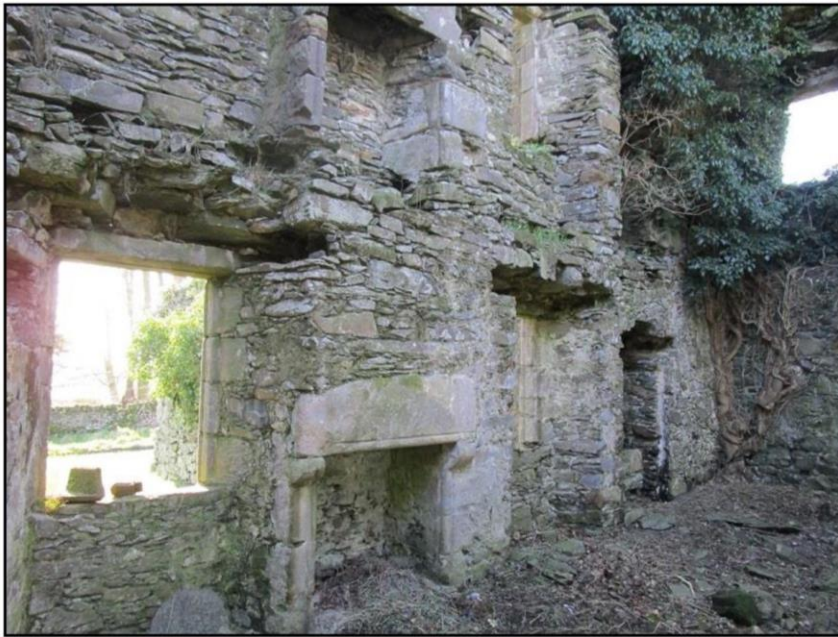
Figure 12: View of NNW-Facing Internal Elevation, with Large Fireplace
