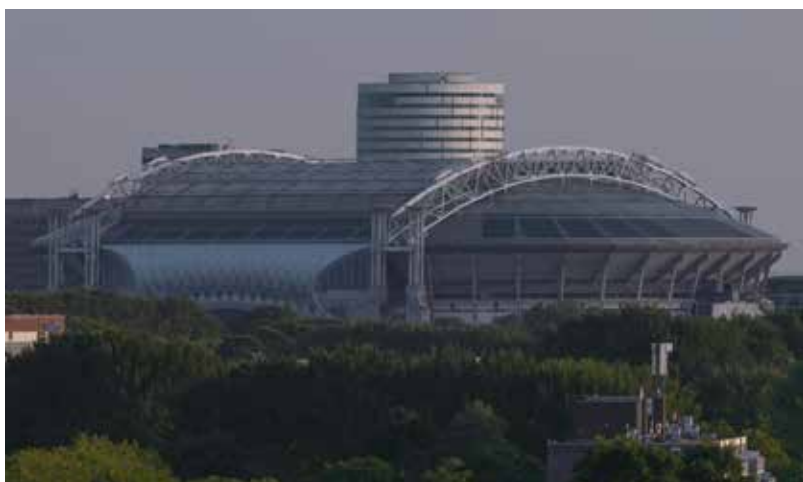
The Johan Cruijff Arena in Amsterdam has Europe's largest energy storage system
