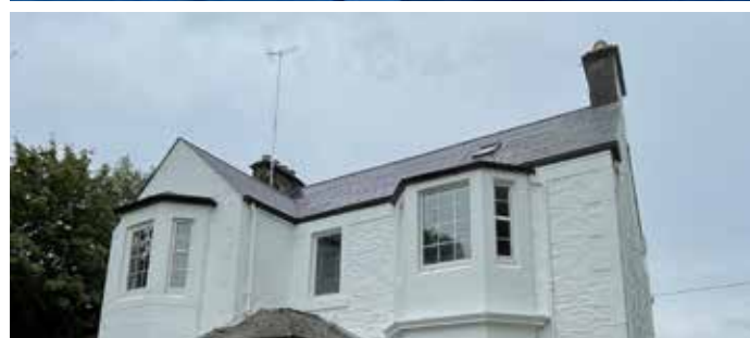
Photos showing solar tiles being fitted and then a finished installation illustrating how they blend in
