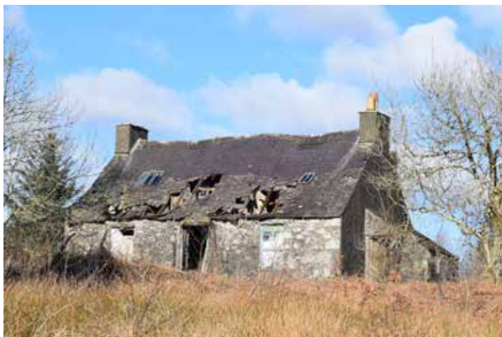
The neglected former holding of Druim an Easa, Castlemaddy Forest; could new life be breathed back into these abandoned crofts?
