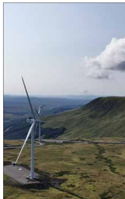
Completed turbines at the Windy Rig Wind Farm
