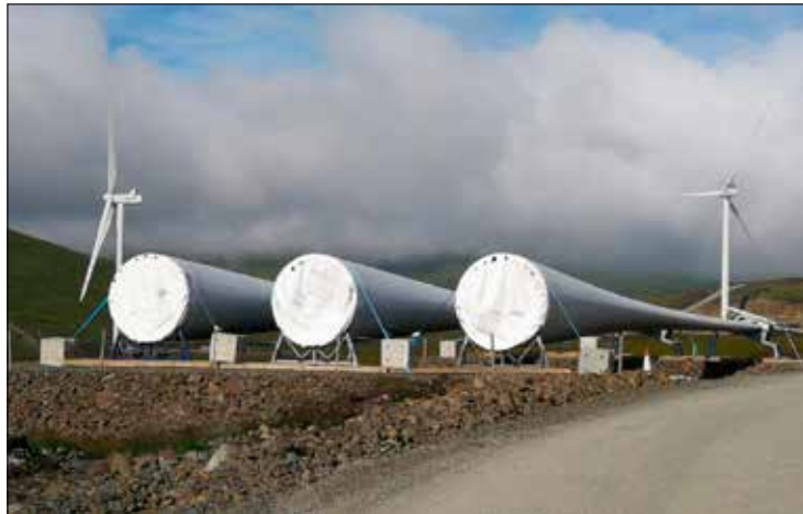
Blades waiting to be lifted into position
