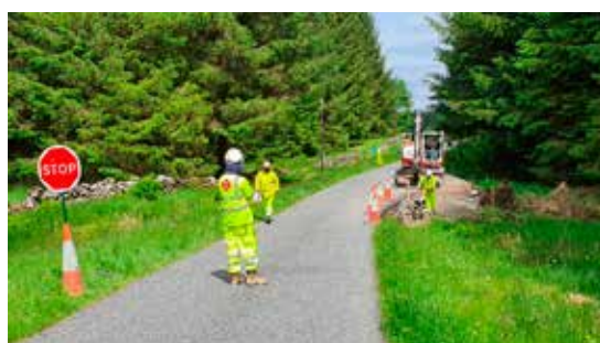
Top: Track construction taking place on the Windy Rig site. Above: Passing place construction along the B729.
