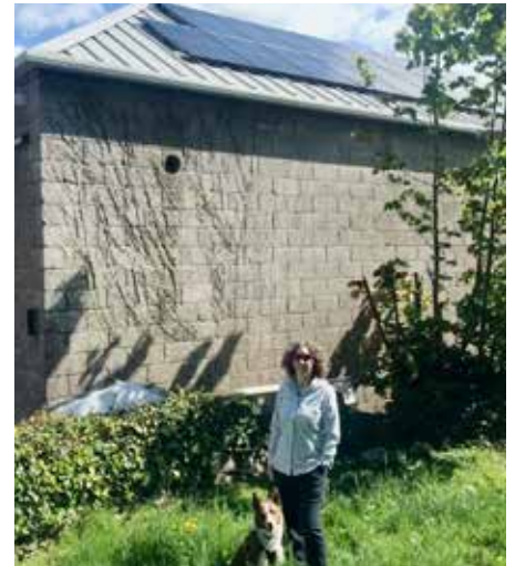
Gill (and Hamish) admiring the new solar PV hard at work in sunny Balmaclellan
