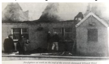
Firefighters at work on the roof of the severely damaged Killisnoe Hotel
