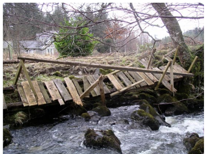
Top: repairing the bridge. Above: the bridge with the schoolhouse is visible in the background.
