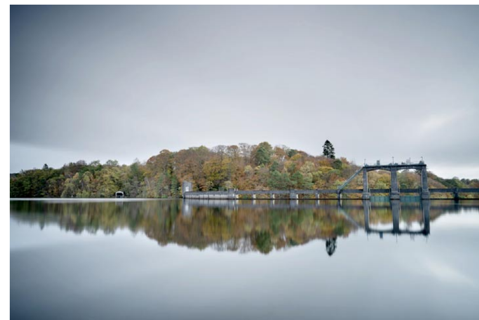
Earlstoun dam, part of the Galloway hydro electric scheme.
