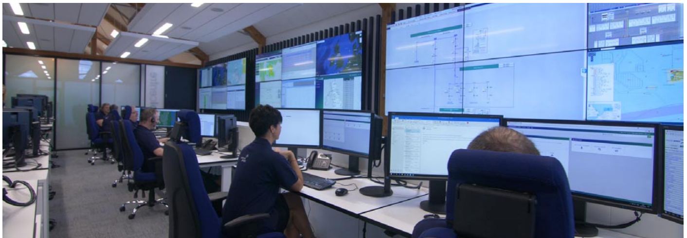
The new ControlCentre at The Green House, Forrest Estate, Dalry.
