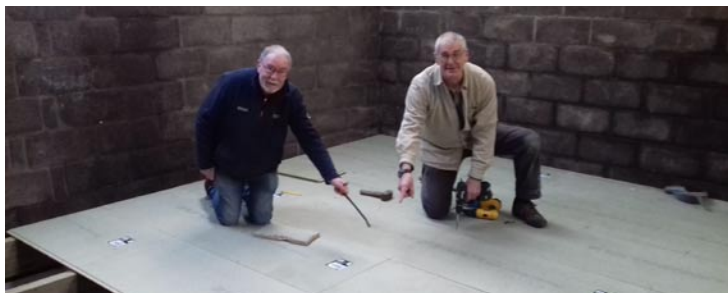
Ali Stewart and Stuart Rhodes working on the mezzanine floor at the Men's Shed.
