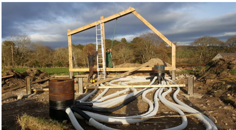
Pictures: Top - Preparing 'hugel beds' with logs, manure, pond weed, seaweed and soil; Below - Pipes laid for the passive solar underfloor heating in the green house; Right - Lorraine harvesting from her no-dig 'lasagne bed'.
