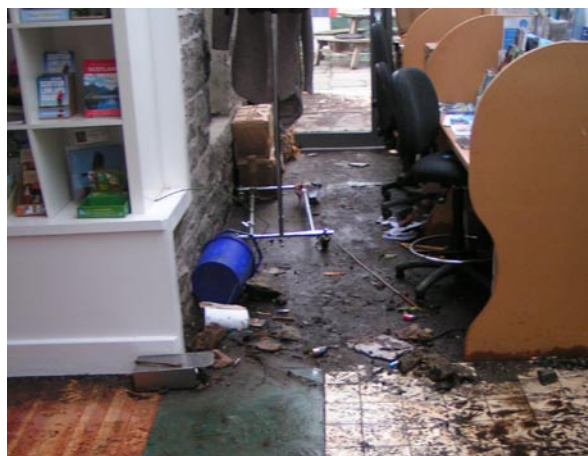
Flood damage in the hallway by the computer desks in the CatStrand.
