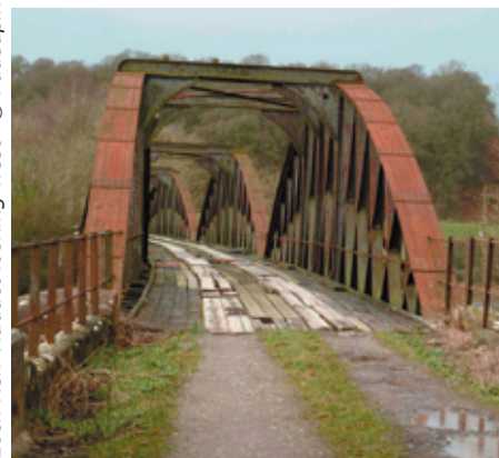
Loch Ken Viaduct looking west- © Padeapix
